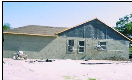
Stucco being installed on model house
