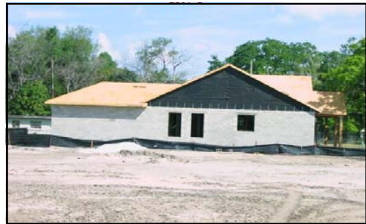
Model house construction
