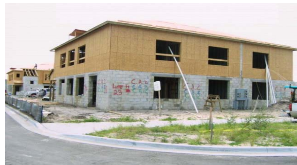
Construction on the quad units is underway.
